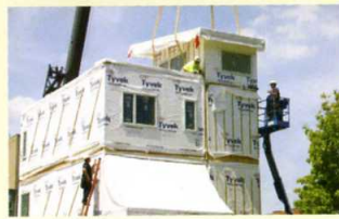
Above: Modular components of the downtown Dayton Litehouse project are pre-built then assembled onsite, helping to reduce wasted construction materials sent to the landfill.
