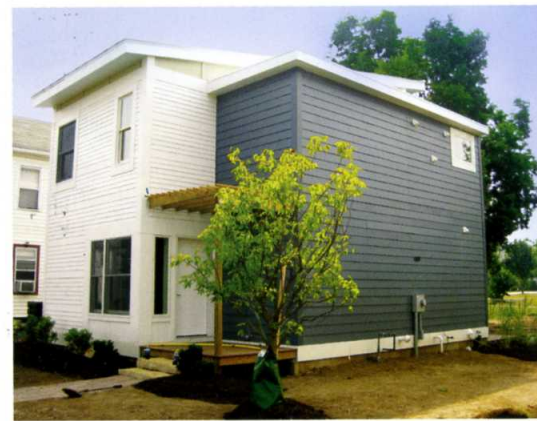
Nearly complete, state-of-the-art, energy efficient Litehouse Demonstration Home in West Carrollton.
