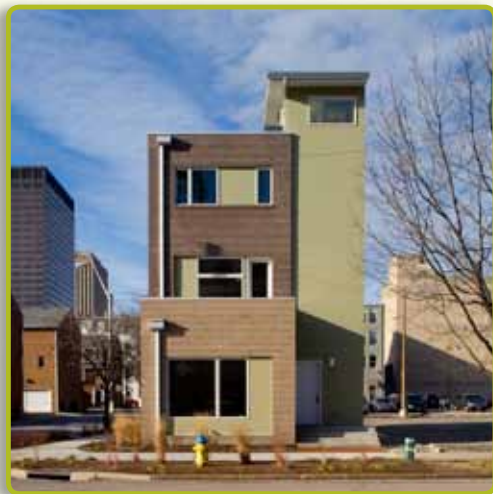
The demonstration Town Home is located at 123 North Patterson Boulevard, Downtown Dayton.
