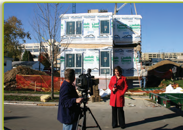
Channel 7 News provided media coverage of the installation.
